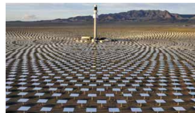
Solar thermal energy
